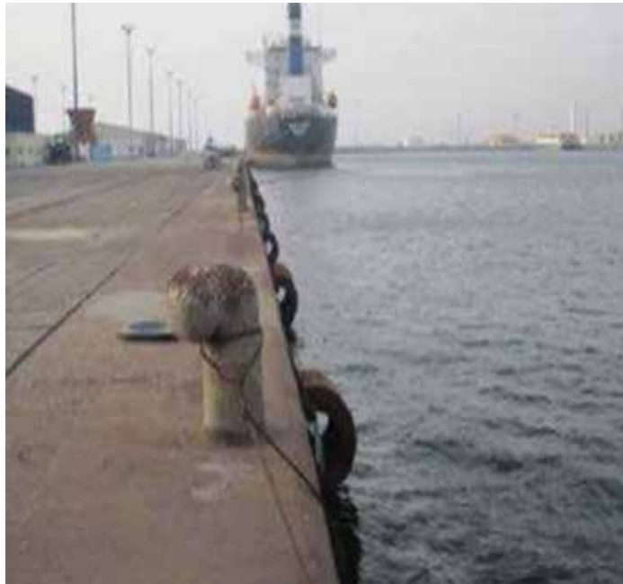
Renovation Of Port Berths
