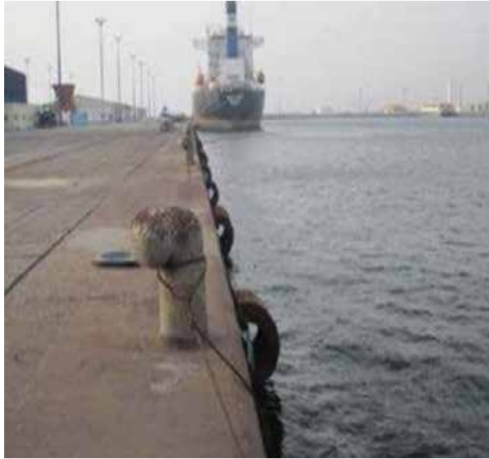
Renovation Of Port Berths
